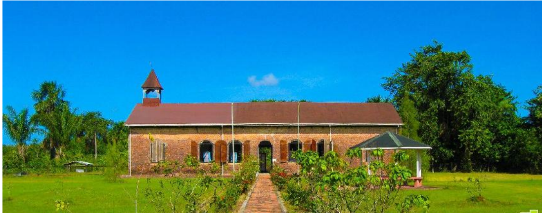
The church on Fort Island
